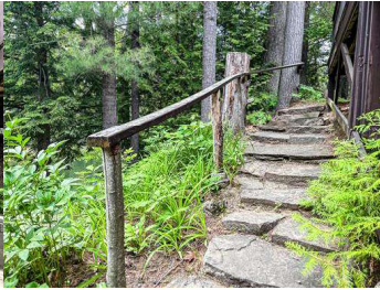
steps to lower patio
