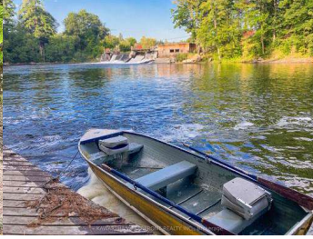
Views of the Norland Dam
