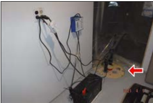
5.5 Item 3(Picture) Sumppump-alarm-battery
