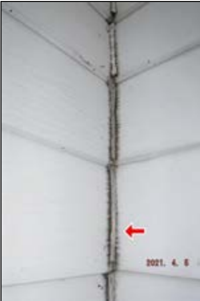
2.6 Item 1(Picture) Caulking failing
