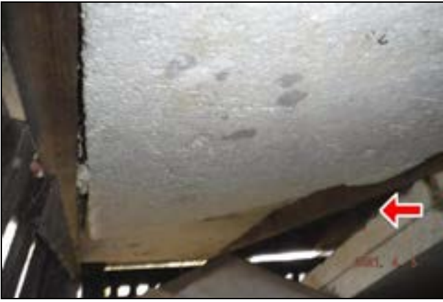
9.3 Item 1(Picture) Foam Board insulation
