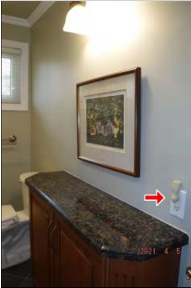
6.6 Item 1(Picture) GFCI protected receptacle
