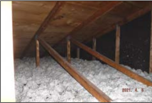
9.0 Item 3(Picture) Cellulose insulation
