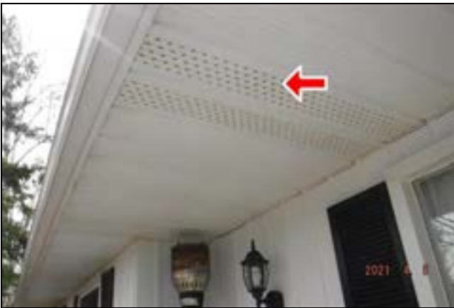
9.1 Item 1(Picture) Soffit venting
