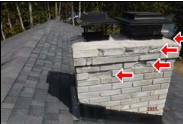
7.2 Item 1(Picture) Failing mortar and brick
