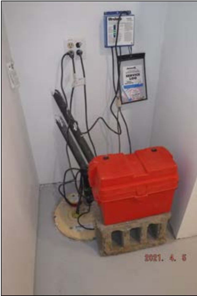
5.5 Item 1(Picture) Sump pump-Battery-Alarm
